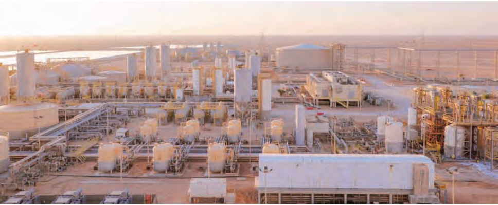
OQGN's pipeline network expanded to 4,368 kilometres in 2025, an increase of 133 kilometres compared to the previous year.
