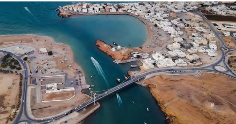
Work is underway on 158 projects within the governorate's programme.
