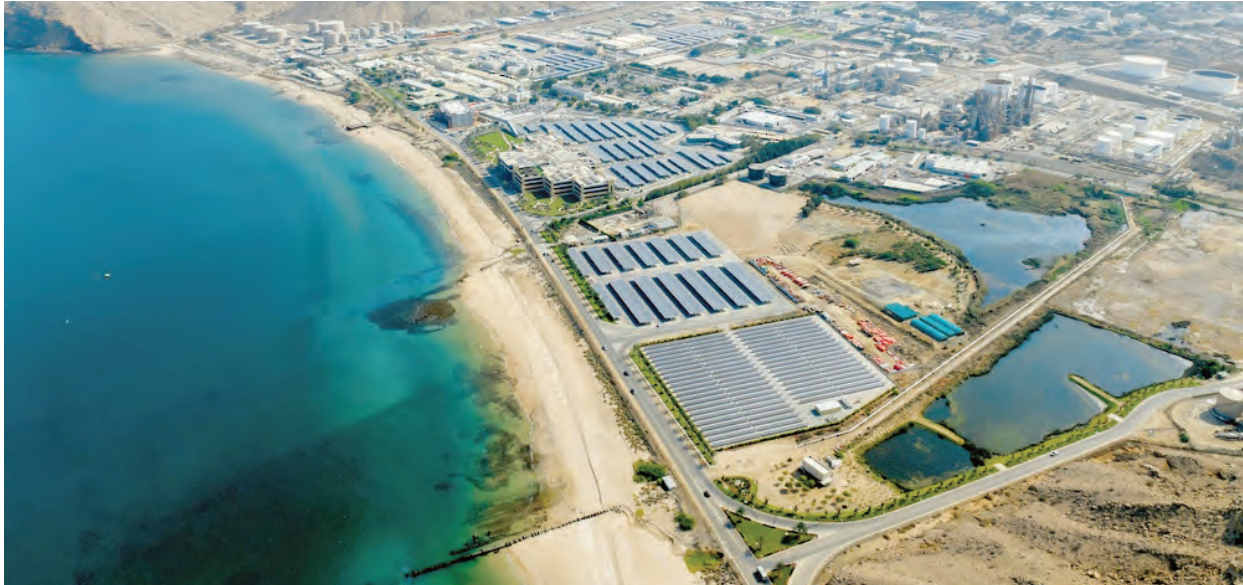
The Integrated Operations Centre at Bait Al Haitham is designed to unify the remote monitoring and management of PDO’s oil, gas and energy assets within a single integrated operational environment.
