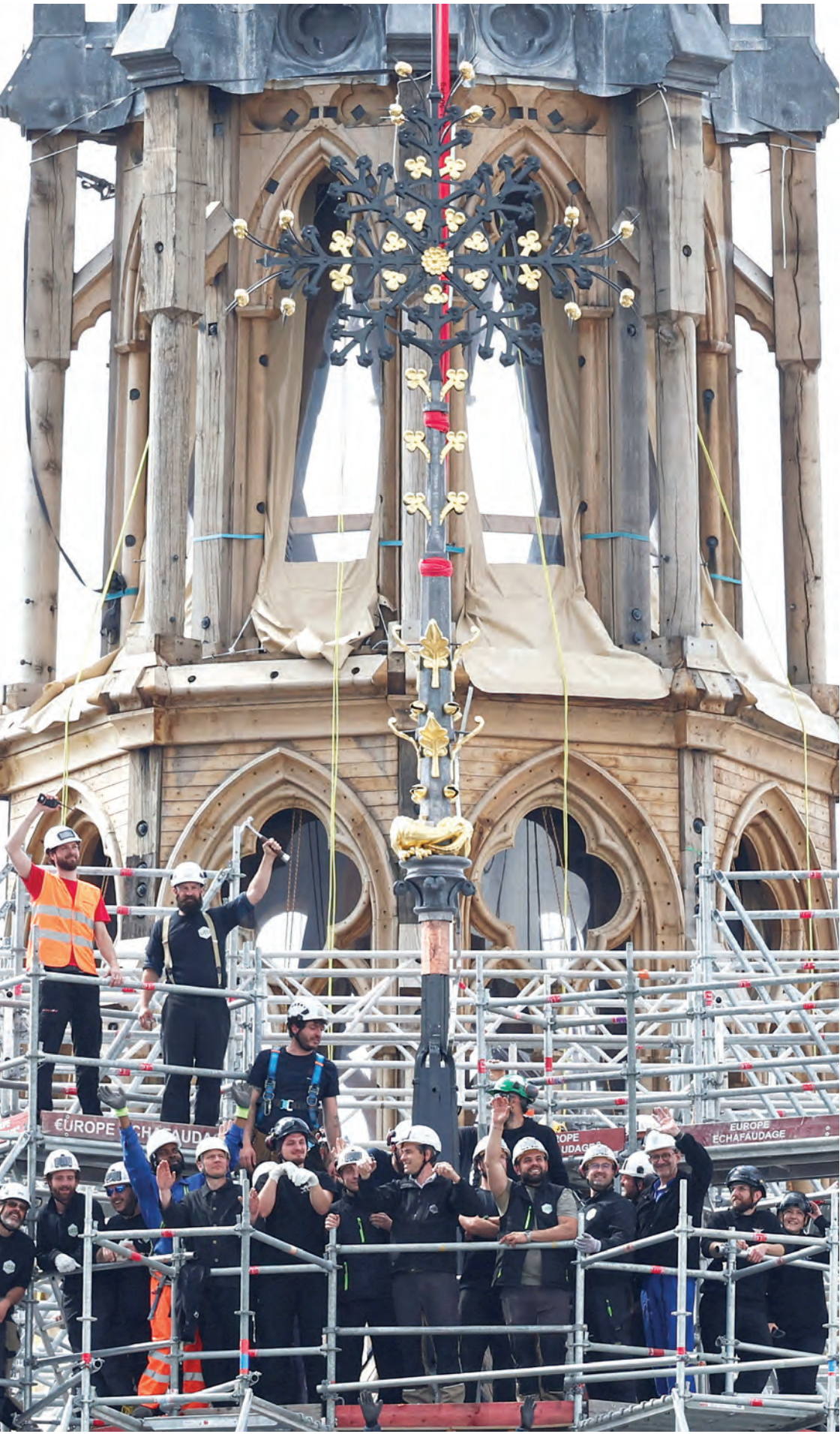
Workers react after a crane installed the restored 'Croix de chevet' cross at the top of the choir of the Notre-Dame de Paris Cathedral, which was ravaged by a fire in 2019, as restoration works continue in Paris, France, on Saturday. – Reuters
