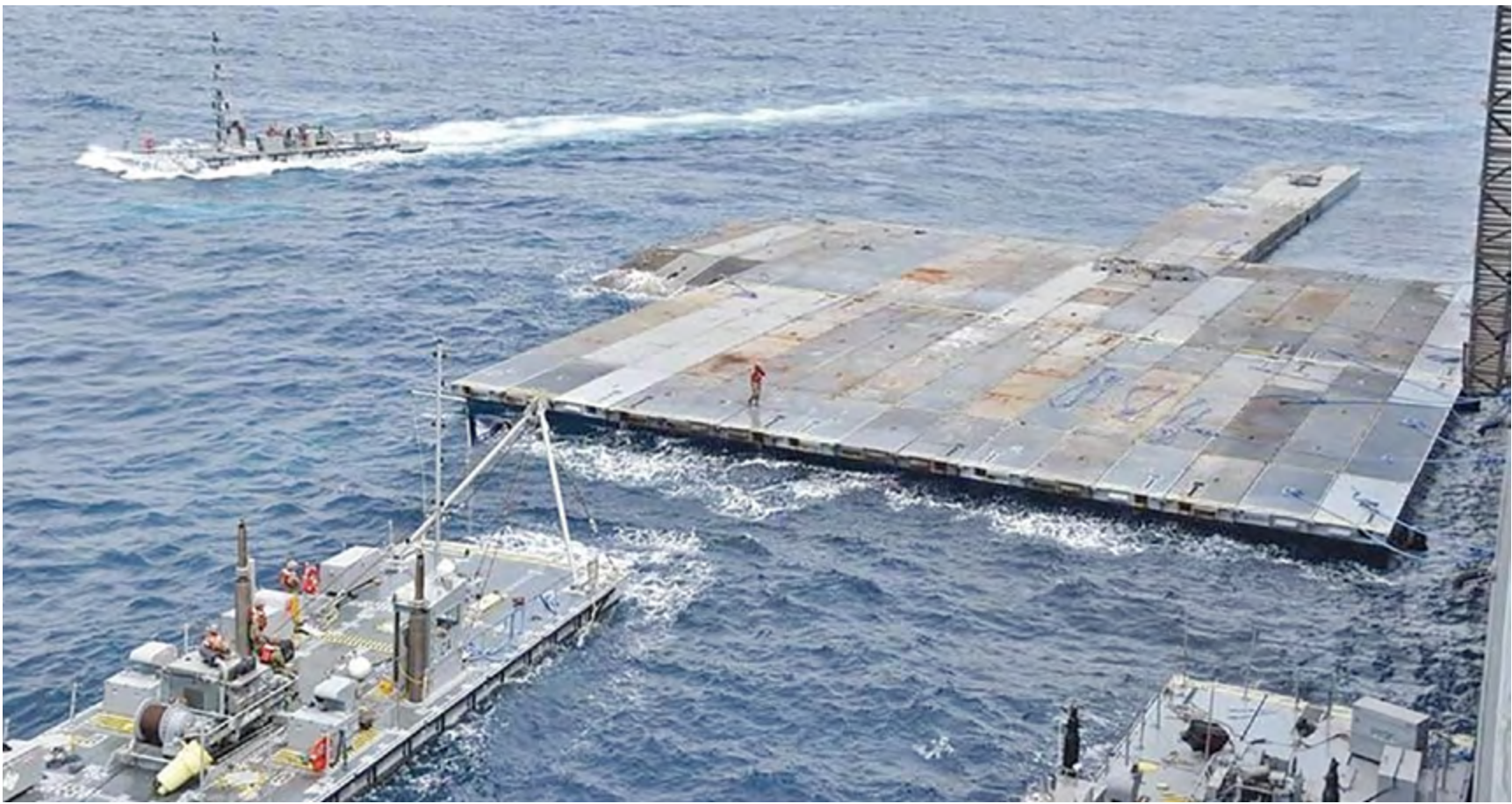
Since the pier became operational on May 17, more than 8,100 metric tonnes of humanitarian aid has been delivered to the marshalling area for onward delivery and distribution
