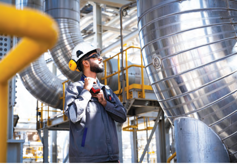
A key part of OQ8’s success has been its ability to optimise refinery capacity without major modifications.
