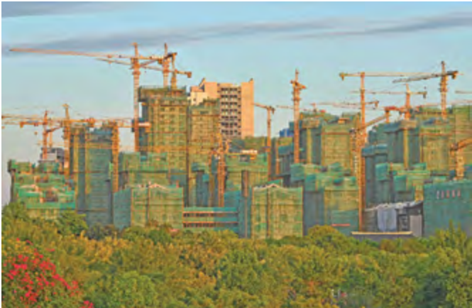
A residential complex is seen under construction in China (AFP)
