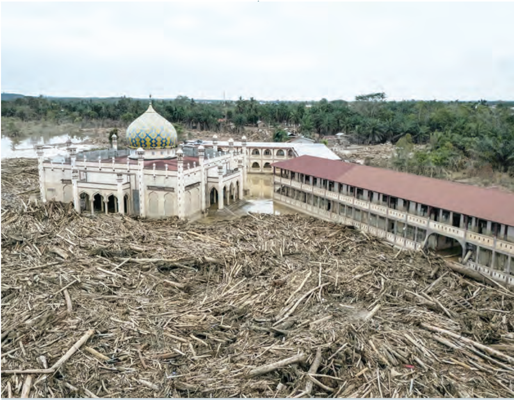
An aerial view shows piles of uprooted trees swept away by a flash flood about three weeks ago at Darul Mukhlisin Islamic Boarding School and the mosque attached to the school in Aceh Tamiang, Northern Sumatra. — AFP
