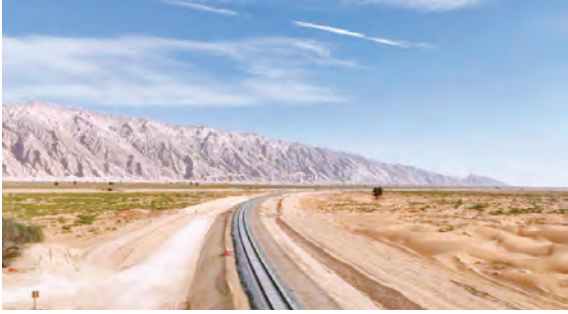
The Hafeet Rail project has now transitioned from excavation and civil construction to the rail infrastructure construction phase.
