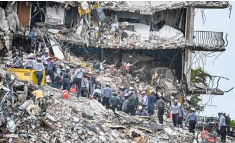
Search and rescue teams look for possible survivors in the partially collapsed 12-story Champlain Towers South condo building on Tuesday in Surfside, Florida. – AFP
