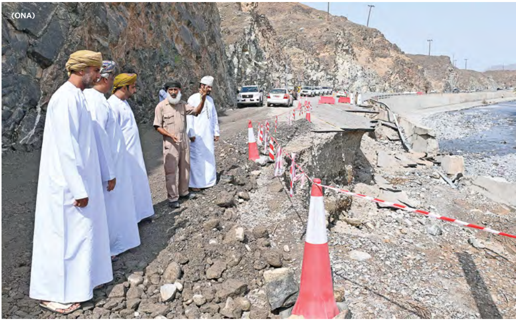
MTCIT Undersecretary H E Dr Ali al Shedhani inspects restoration of a road along a wadi in the Falaj Bani Khazir
