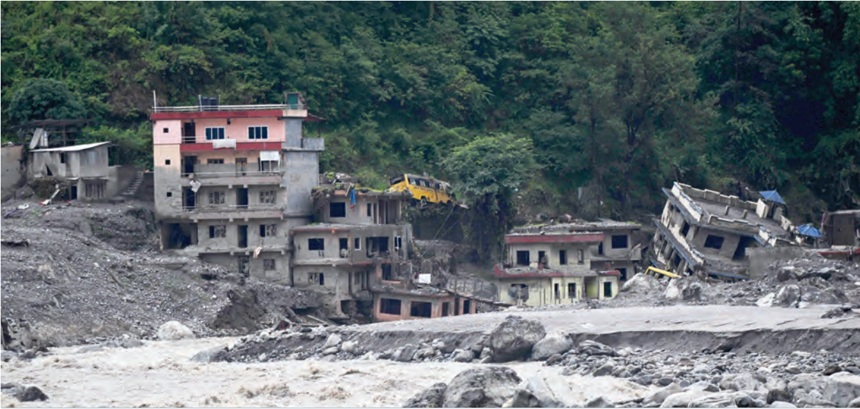
A general view shows damaged houses covered in sludge in the aftermath of the August 26 flash flood at Betrawati Bazaar in Nepal's Rasuwa district. — AFP
