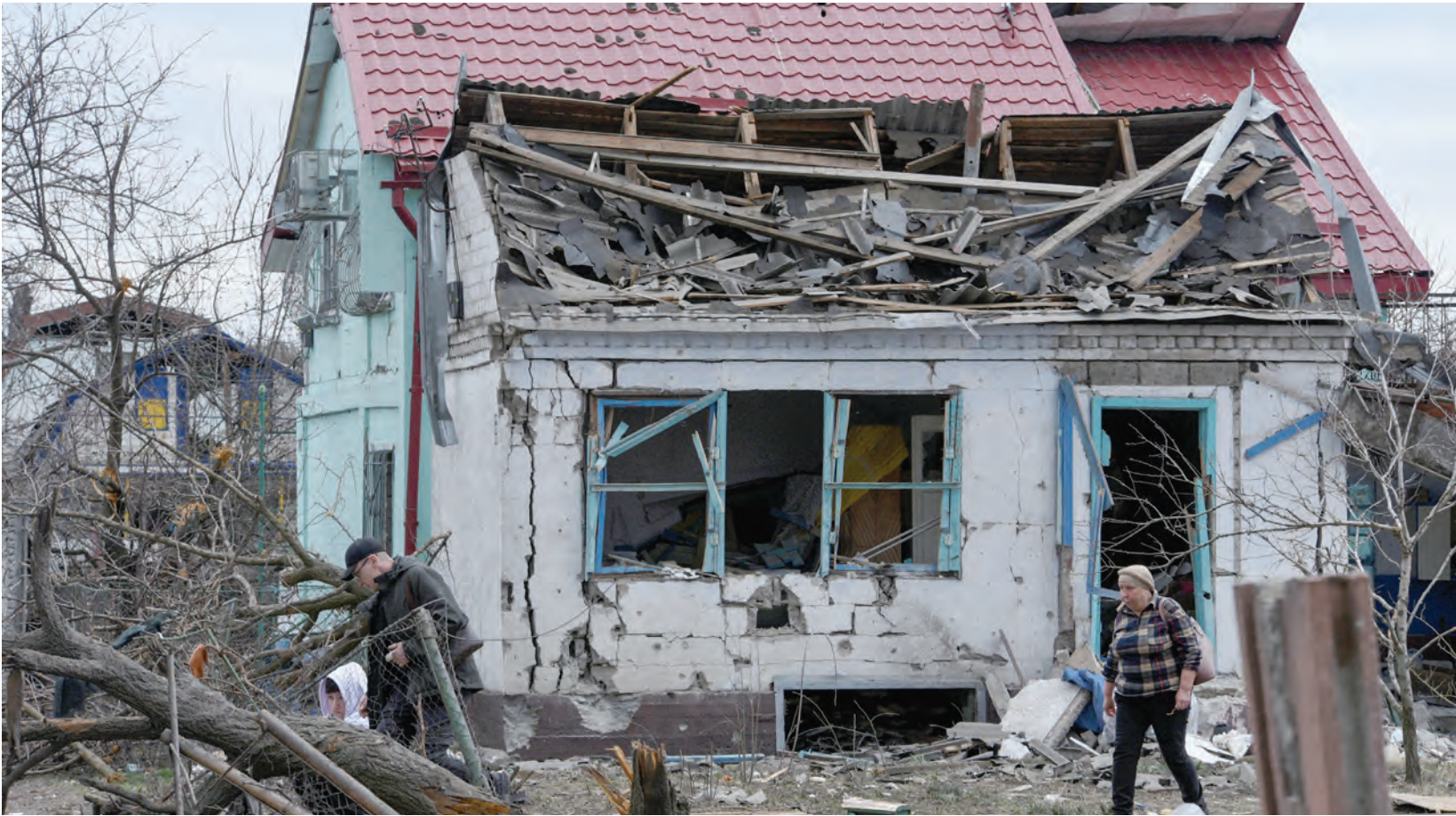
Local residents walk next to their house damaged during a Russian missile and drone strike, in the city of Kamianske, Dnipropetrovsk region, Ukraine. — Reuters
