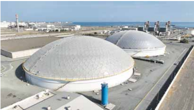
One of the key initiatives is the water transmission project from Suhar's desalination plant to Al Dhahirah Governorate, at a cost exceeding RO 150 million.
