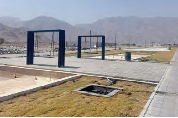
The project is being implemented to transform it into a recreational destination. — ONA
