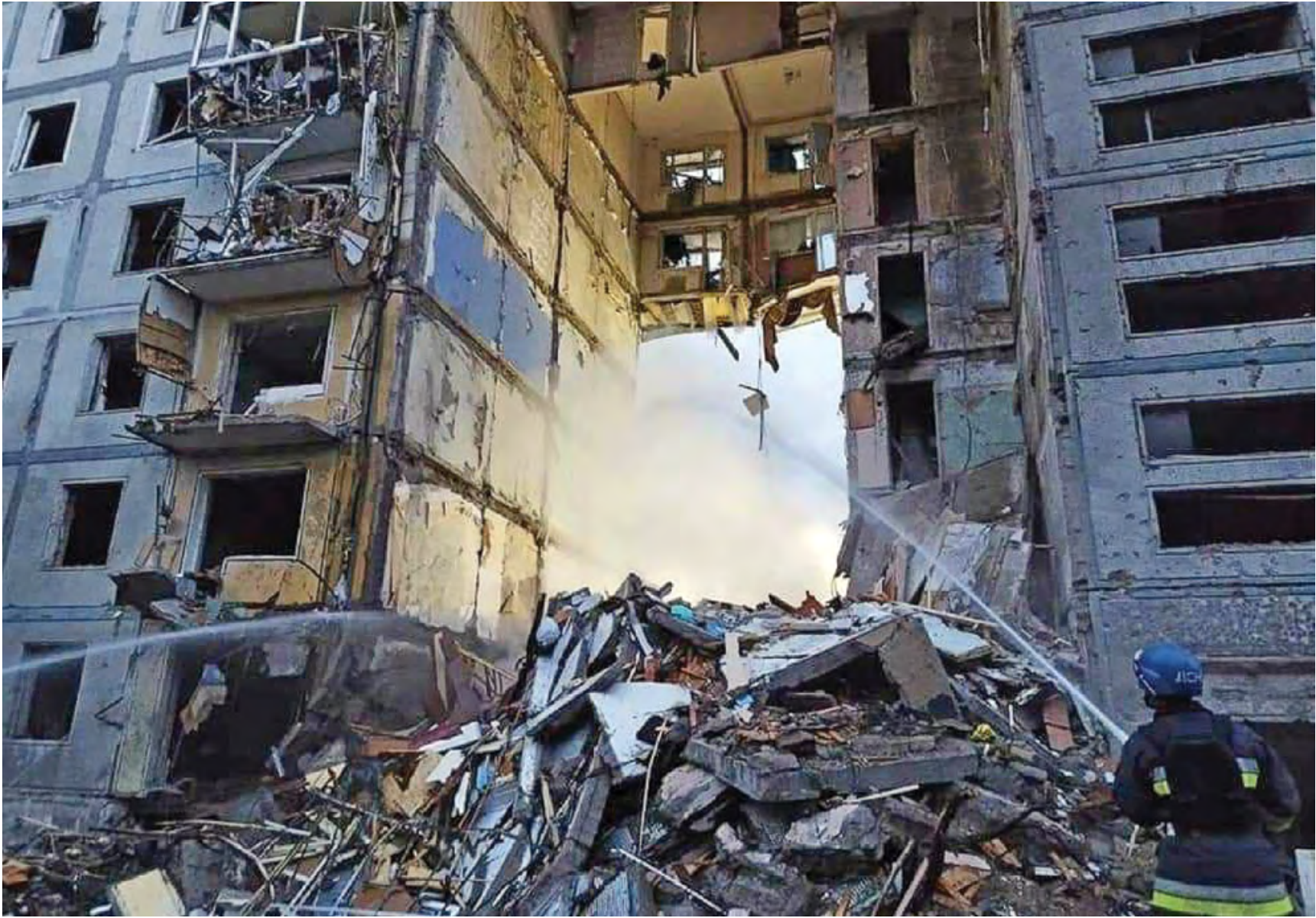
A rescuer with a hose extinguishes a fire in a residential building damaged after a strike in Zaporizhzhia on Sunday (AFP)
