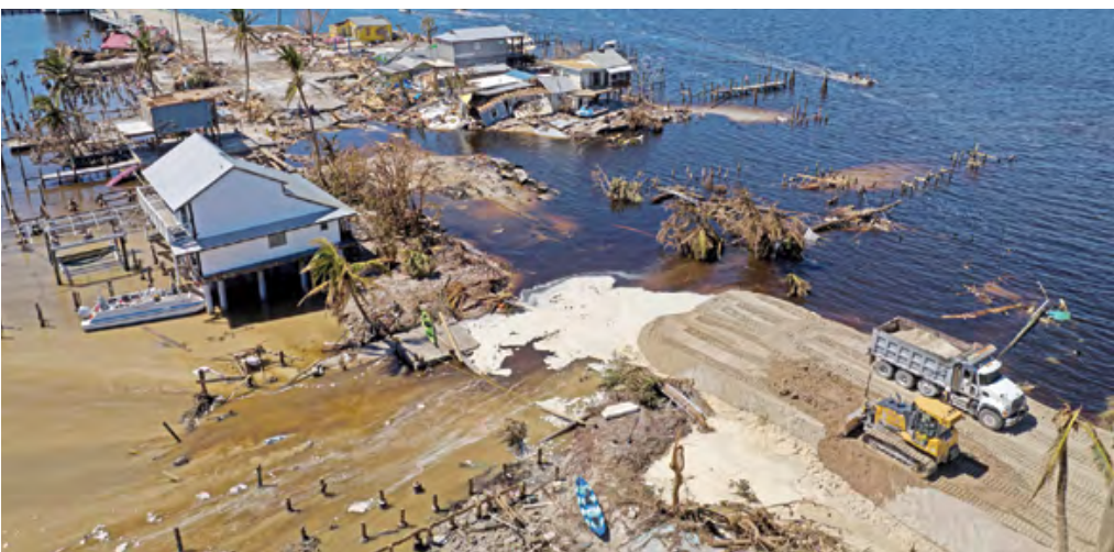
This file photo shows a dump truck dumping its load during emergency repairs to restore road access in the aftermath of Hurricane Ian in Matlacha, Florida on October 03 (AFP)
