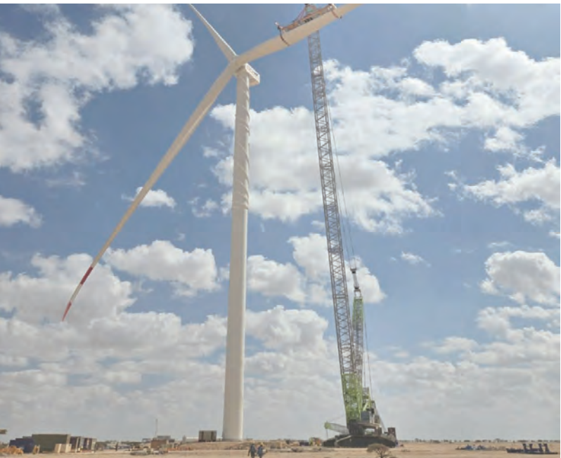
First wind turbine supplied by Goldwind being hoisted at the Riyah-2 site in PDO’s concession
