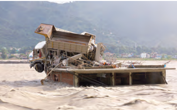
A flooded home, with damaged trucks on its roof, along the banks of the Trishuli River, following the deadly flash floods and mudslides in Nuwakot district, Bagmati province, Nepal. — Reuters
