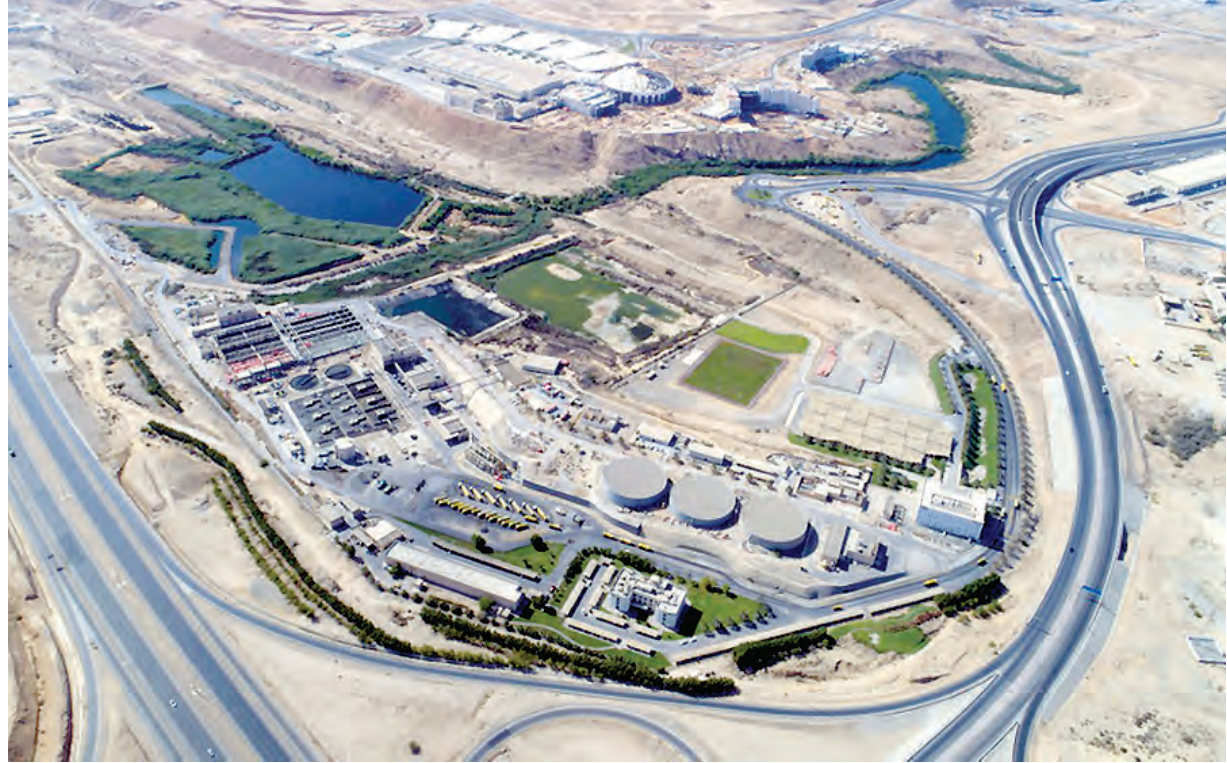
Sewage network and treated water in the Bawshar area (B8)
