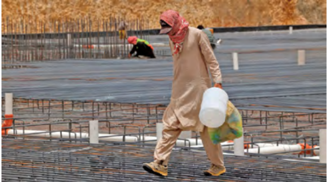
This file photo shows a labourer walking with an empty water container at a construction site in Saudi Arabia's capital Riyadh on May 23, 2022 (AFP)
