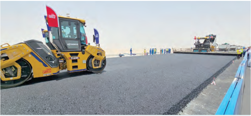
The launch represents the development of roads and automation of construction projects.
