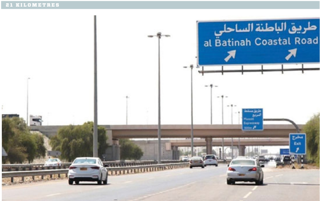
TWO-WAY ROADS: As part of the project, two-way roads will be constructed along Al Batinah Expressway and connect the economic zone of Khazaen and the overall national road grid. - ONA
