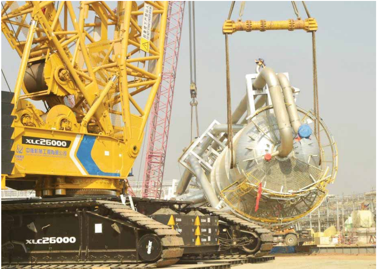
Super-heavy equipment being installed in Bangladesh's largest fertilizer factory A carbon dioxide stripper tower is installed at a fertilizer plant under construction in Narsingdi, Bangladesh, on Tuesday. The carbon dioxide stripping tower, the first super-heavy equipment of Bangladesh's Ghorashal-Polash Urea fertilizer project (GPUFP), the country's largest and first ever green fertilizer factory, was installed successfully on Tuesday. Xinhua
