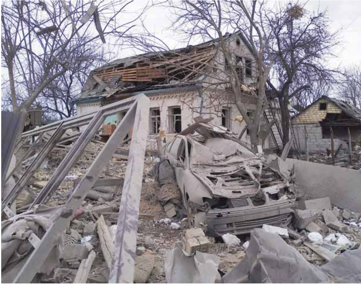
A destroyed car is seen in front of a house damaged by shelling during Ukraine-Russia conflict in the village of Marhalivka in the Kyiv region. – Reuters
