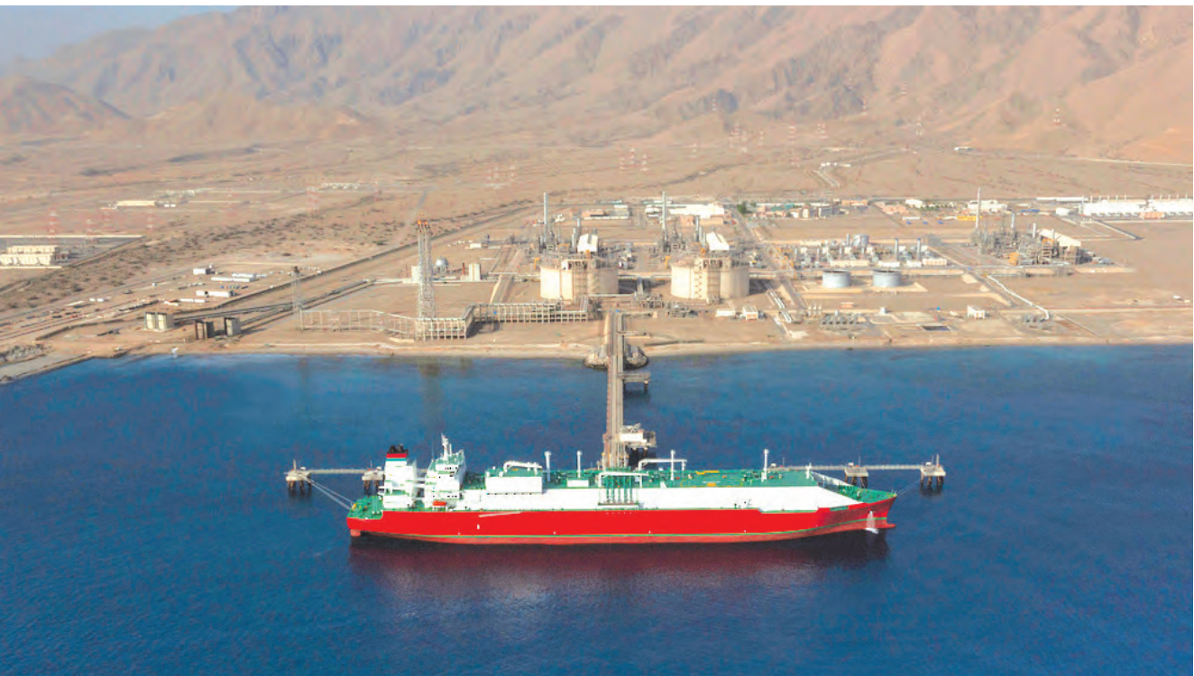
The deployment of Muscat LNG expands Oman’s LNG shipping capacity and reflects closer collaboration between the country’s energy, maritime and logistics sectors.
