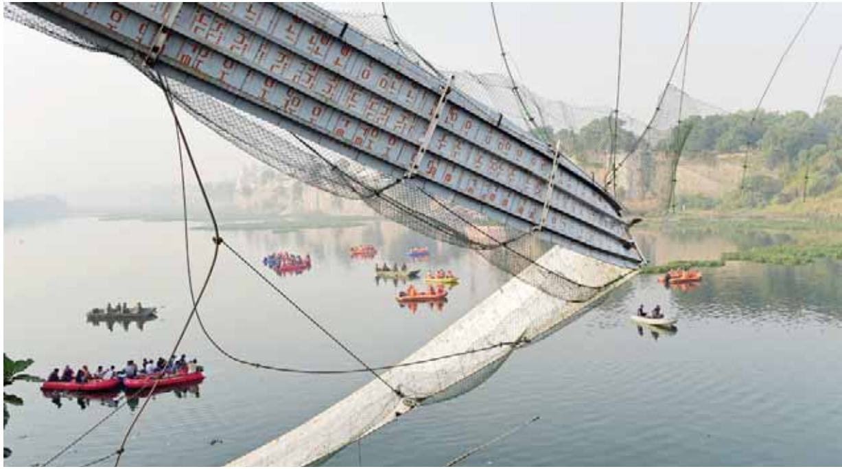
Rescue personnel conduct search operations after a bridge across the river Machchhu collapsed at Morbi in Gujarat on Monday. — AFP
