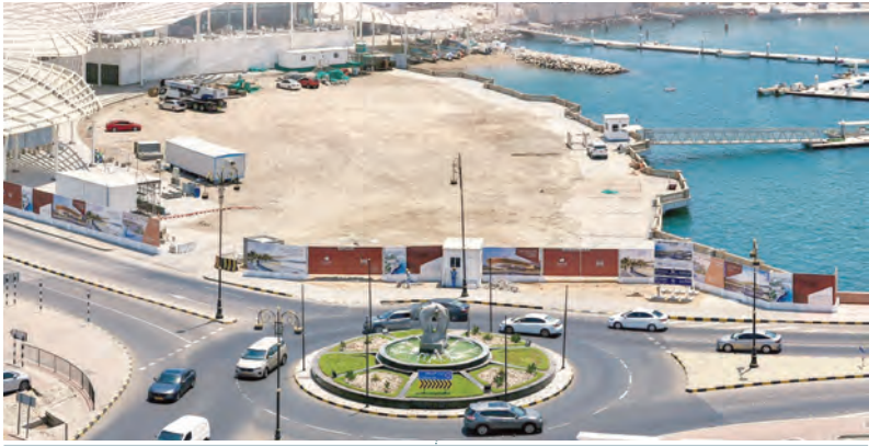
Once complete, Muttrah Square is expected to become a prominent architectural and tourism landmark in the capital.
