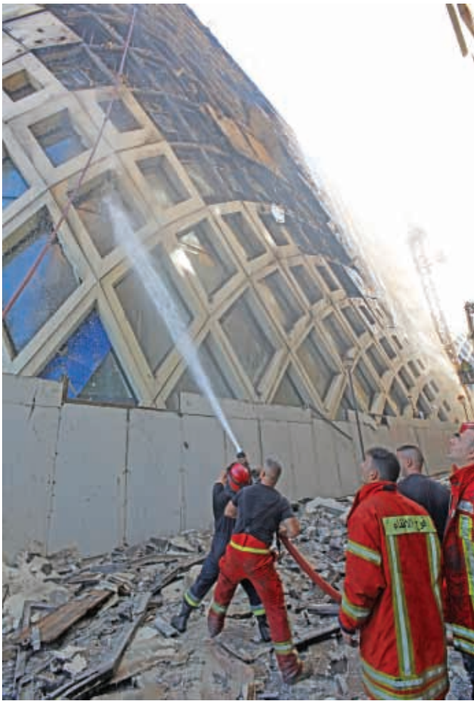
Lebanese firefighters douse the flames of a blaze that engulfed a landmark building, in central Beirut on Tuesday (AFP)
