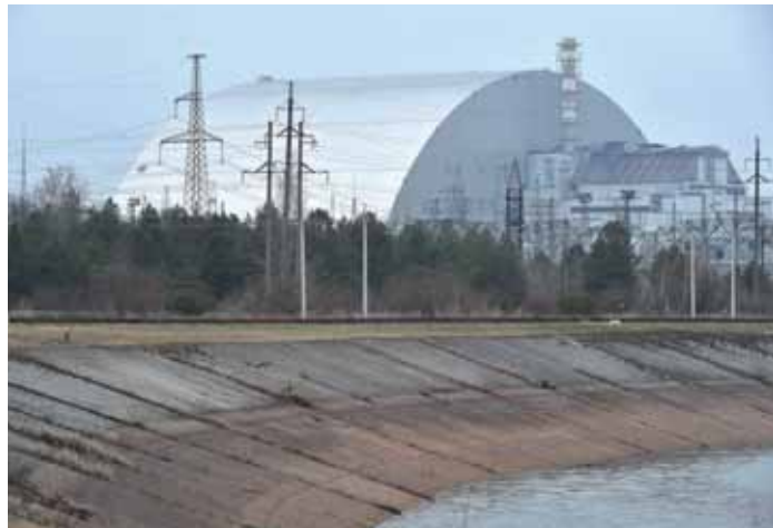
The giant protective dome built over the sarcophagus covering the destroyed fourth reactor of the Chernobyl Nuclear Power Plant — AFP
