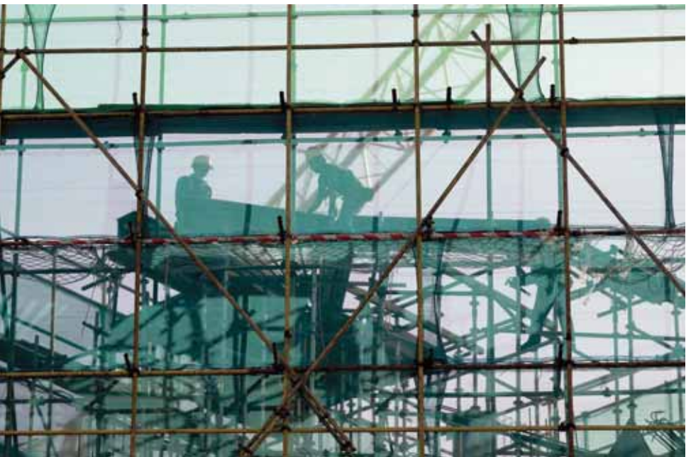
Workers work at a construction site in Beijing. – AFP
