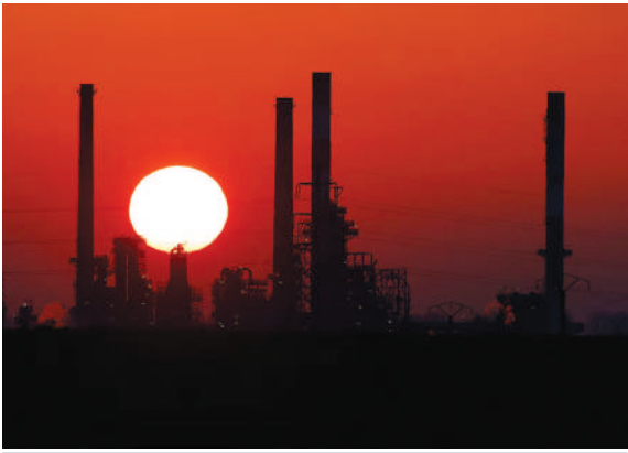
The sun sets behind the chimneys of the Total Grandpuits oil refinery, southeast of Paris, France. — Reuters
