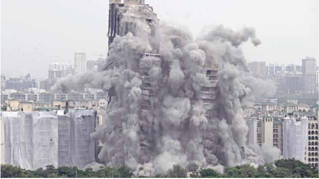
A controlled implosion demolishes the 100-metre-high residential 'Twin Towers' in Noida on the outskirts of New Delhi. — AFP
