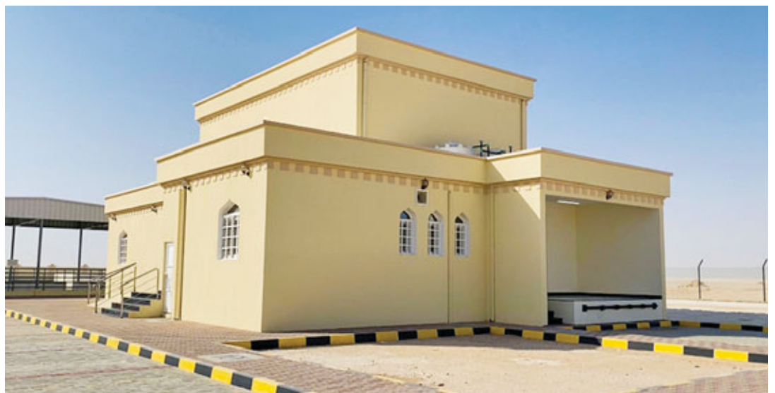
SUSTAINABLE DEVELOPMENT: The projects were funded by PDO as part of its Social Investment programme to benefit communities and boost sustainable development across the Sultanate. - Supplied picture
