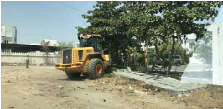
DEMOLITION DRIVE: The Muscat Municipality has decided to remove illegal possessions.
