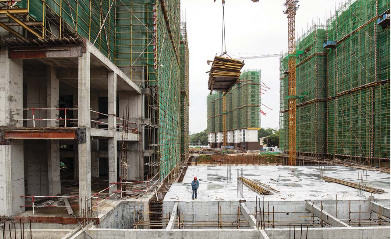
Construction on a residential development in Nanchang, China. – The New York Times
