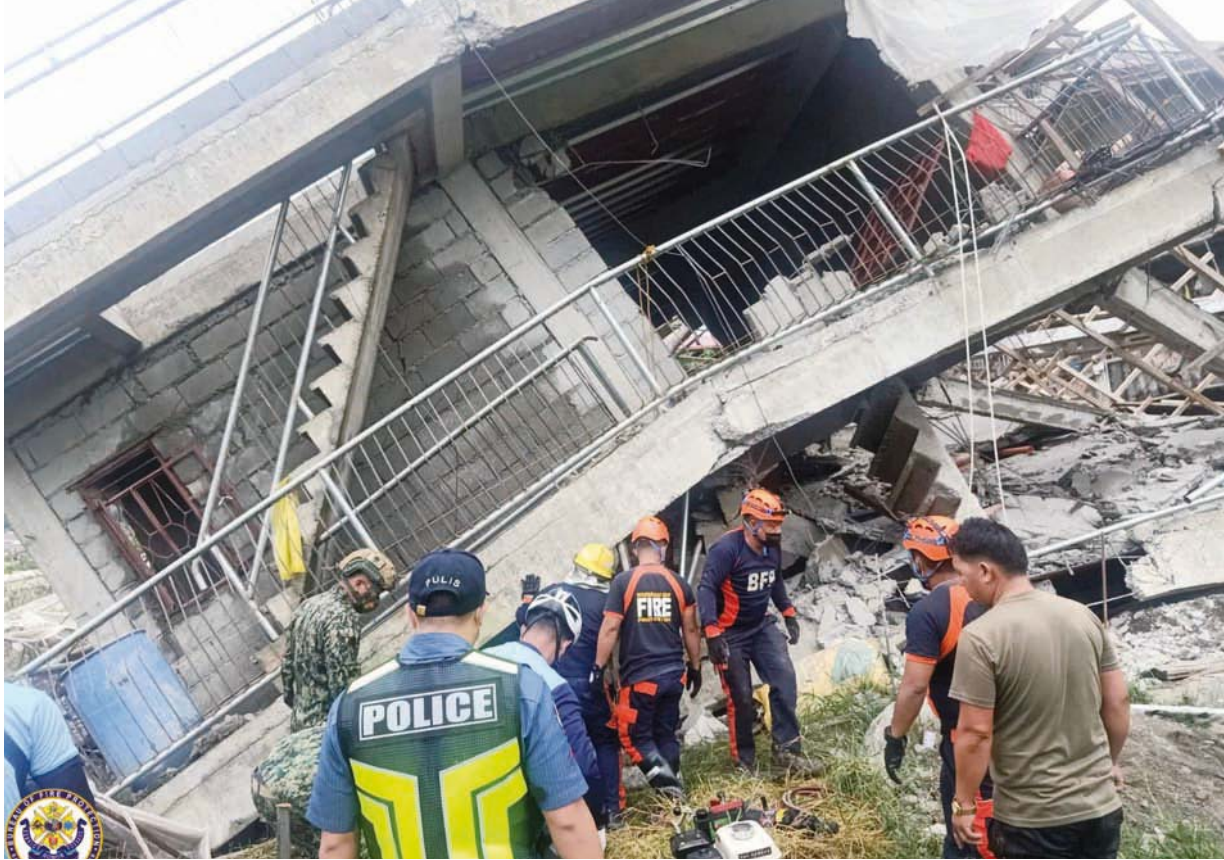
Emergency crew conduct rescue operations outside a building that collapsed during the earthquake, in La Trinidad, Benguet, Philippines on Wednesday. – Reuters
