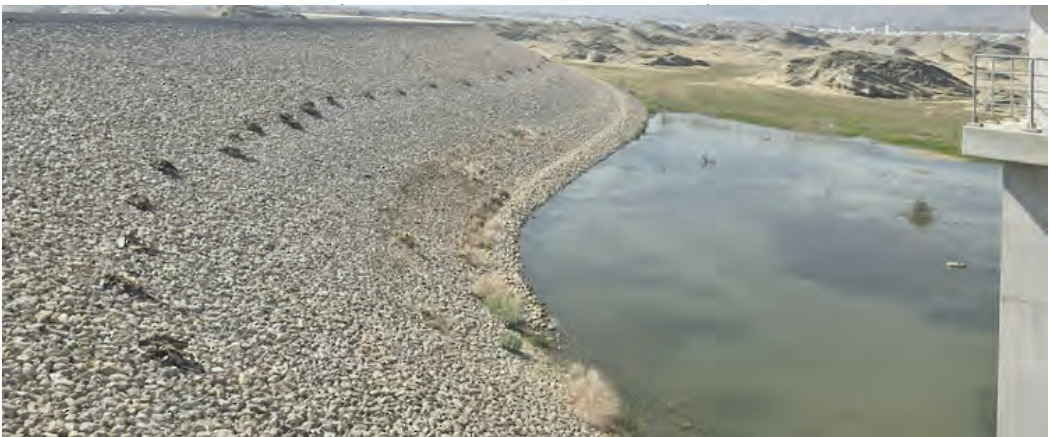
The work aimed to restore the dams’ storage capacity of 13.39 million cubic metres
