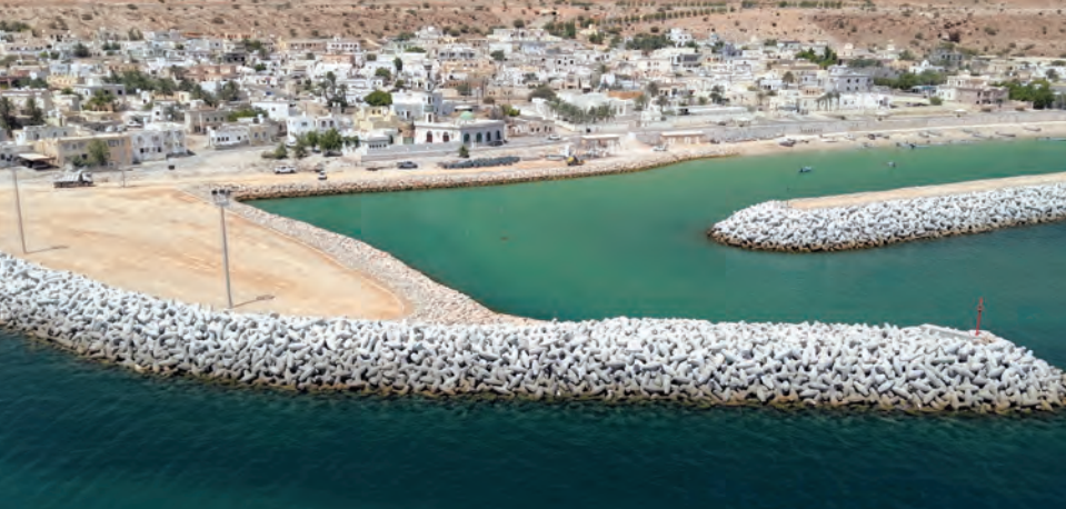
The rehab project enhances infrastructure readiness for the fisheries sector.
