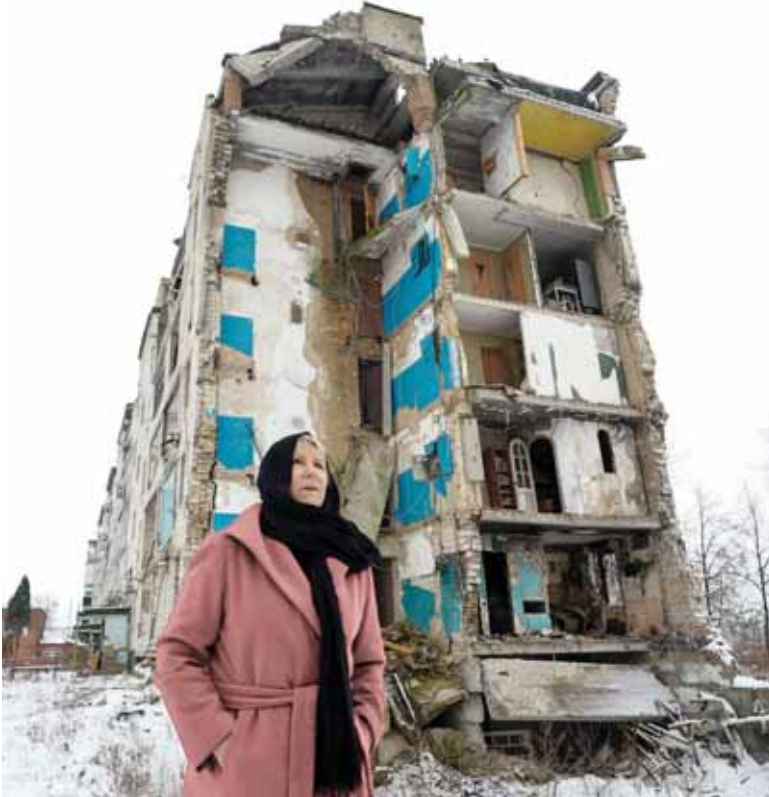
Member of the International Working Group on the Environmental Consequences of War and former Swedish Foreign Minister Margot Wallström stands next to an apartment building heavily damaged during Russia's attack on Ukraine, in the town of Borodianka, Kyiv region, Ukraine. — Reuters
