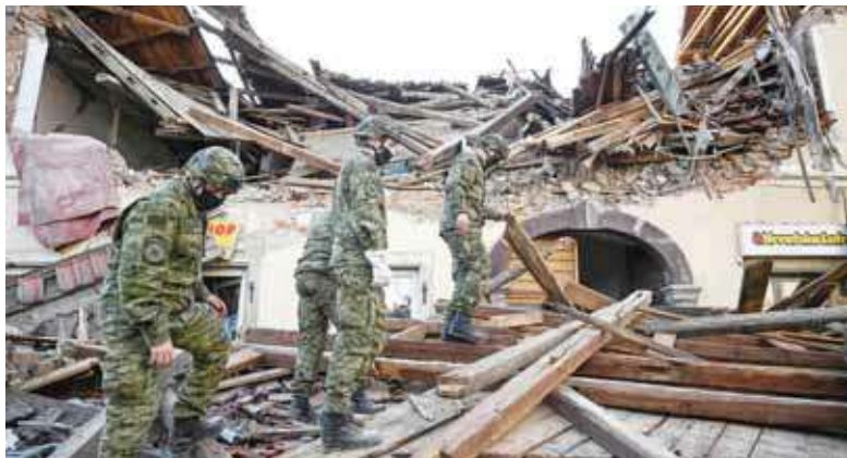
Croatian soldiers walk on wreckage next to damaged buildings in Petrinja, some 50 km from Zagreb, after the town was hit by an earthquake on Tuesday. — AFP
