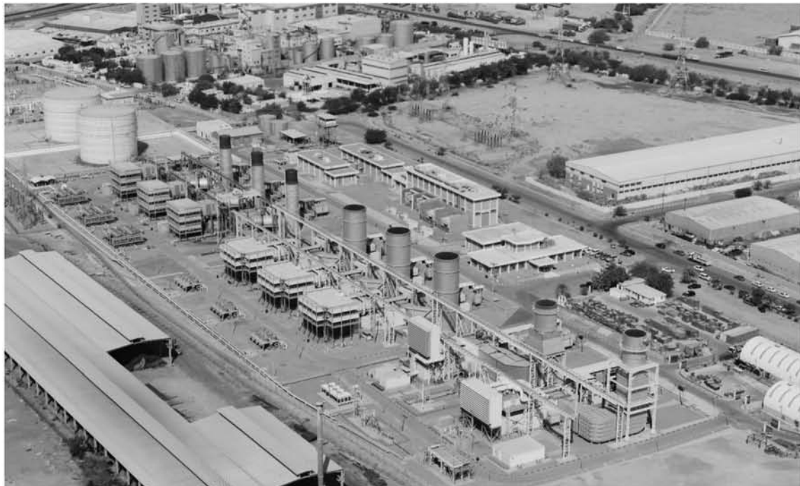
Figure 1 Al Rusail Power Plant
