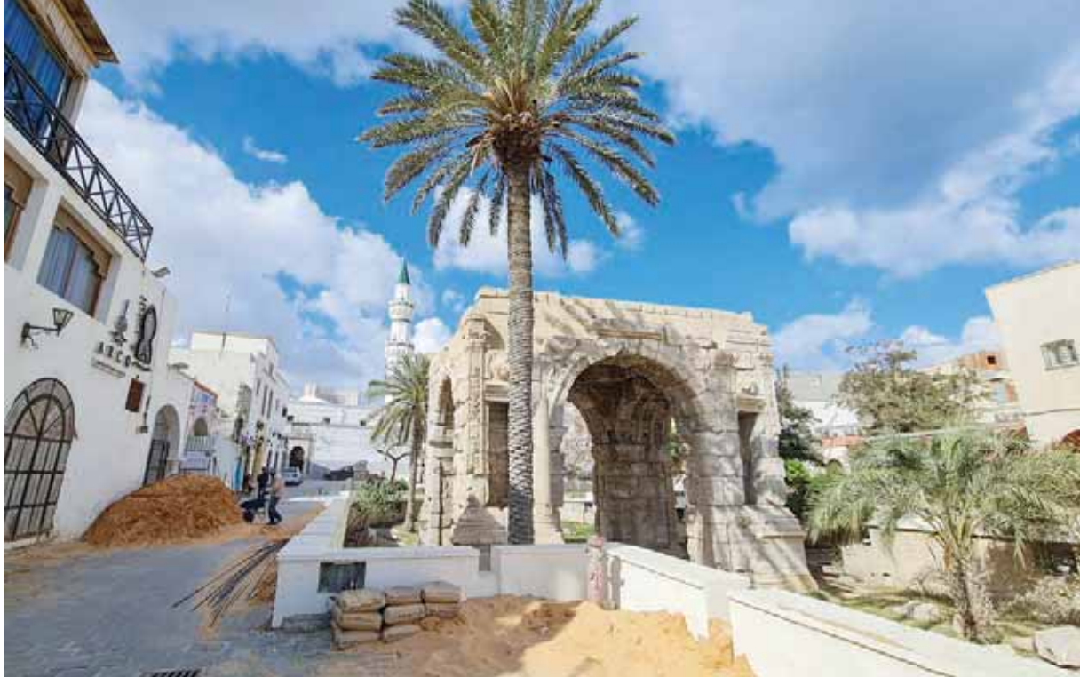
Labourers work on an infrastructure rehabilitation project near the Roman Marcus Aurelius arch in the Libyan capital Tripoli's old city. — AFP
