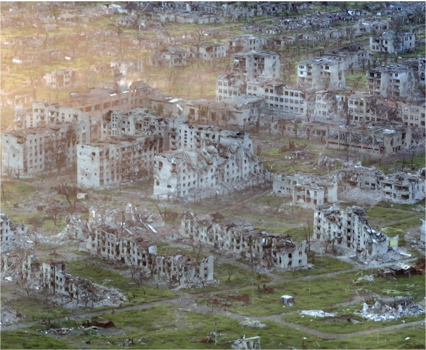
A heavily damaged residential neighbourhood in Marinka, in the Donetsk region of Ukraine.
