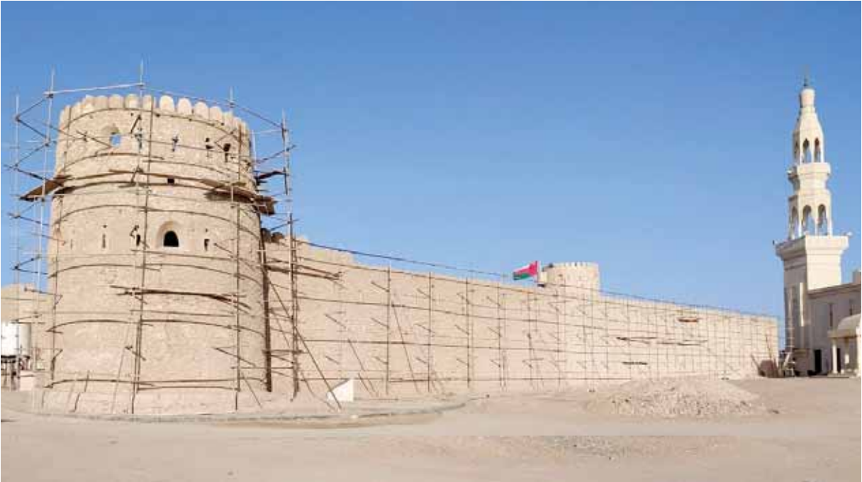
The Ministry of Heritage and Tourism has begun the restoration and maintenance work of the Ras Al Hadd Fort in the Wilayat of Sur. The maintenance work includes rehabilitation to display the holdings, works to remove Al Sarooj mortar and restoration work, treating cracks in the rest of the walls of the fort and the roofs of the western tower and rooms, water leakage works, paving the floor of the outer and inner walls of the fort with flat stones, painting and sanding all wooden materials such as doors and windows, the ministry said. — ONA
