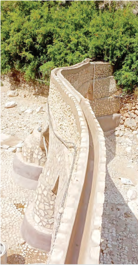
The restoration involved the collection basin and rehabilitating the 150-metre-long channel
