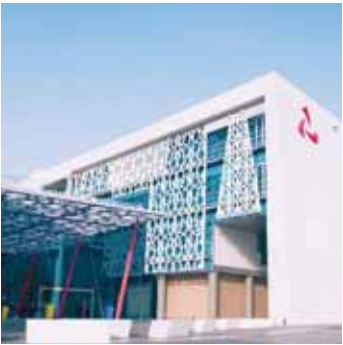
Bank Muscat Facility
