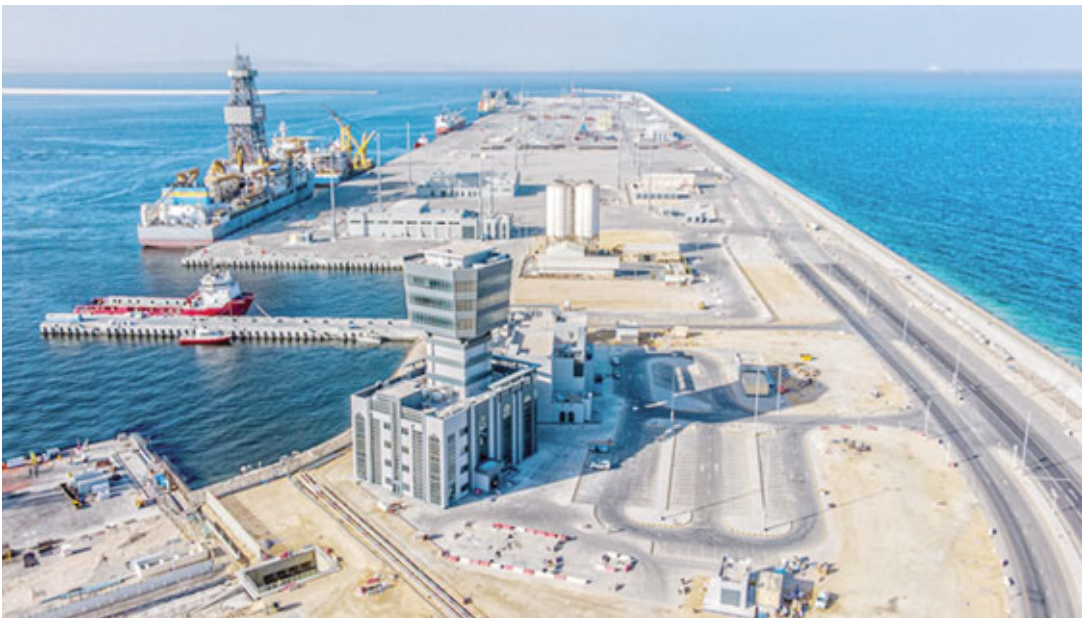
PARTNERSHIP: Asyad Terminals - Duqm, established through a partnership between Asyad Ports and Port of Duqm, will manage and operate three berths in Port of Duqm, which can accommodate the largest container ships and very large crude carriers to serve customers and trade partners. - ONA
