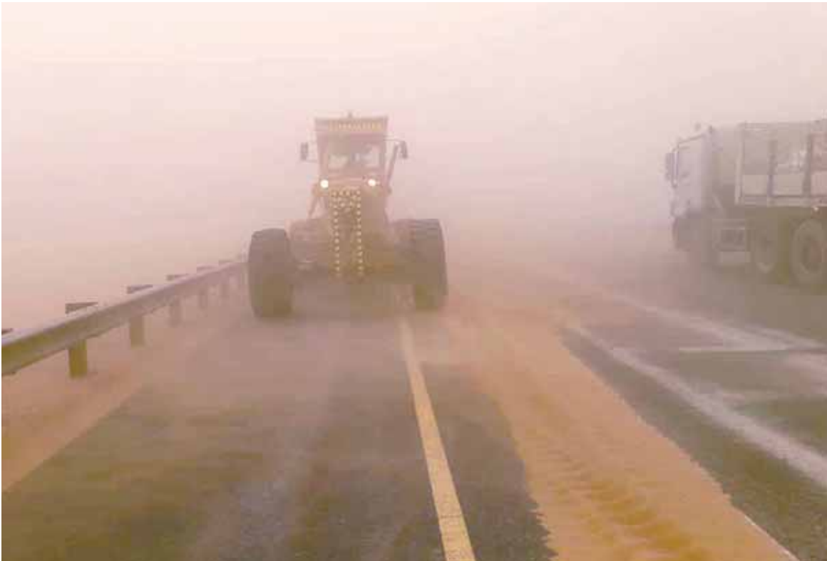
Sand being removed from Adam-Thamrait road.
