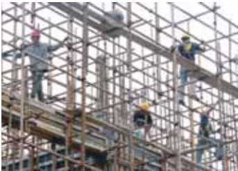
Men work on the scaffolding at a construction site of Hebei Zongheng Iron and Steel plant inside the Tangshan Fengnan Economic Development Zone, Hebei, China. – Reuters
