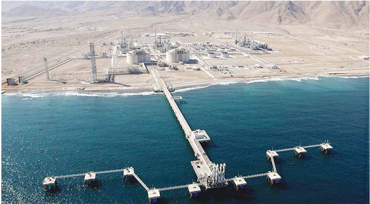
A liquefied natural gas plant is pictured in Qalhat, Oman.
