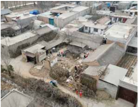
An aerial view shows damaged buildings following the earthquake in Jishishan county, Gansu province, China. — Reuters file photo
