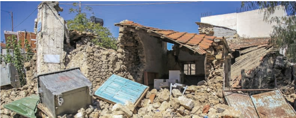
A demolished house following an earthquake, in Arkalochori village on the Crete Island, on Monday (AFP)
