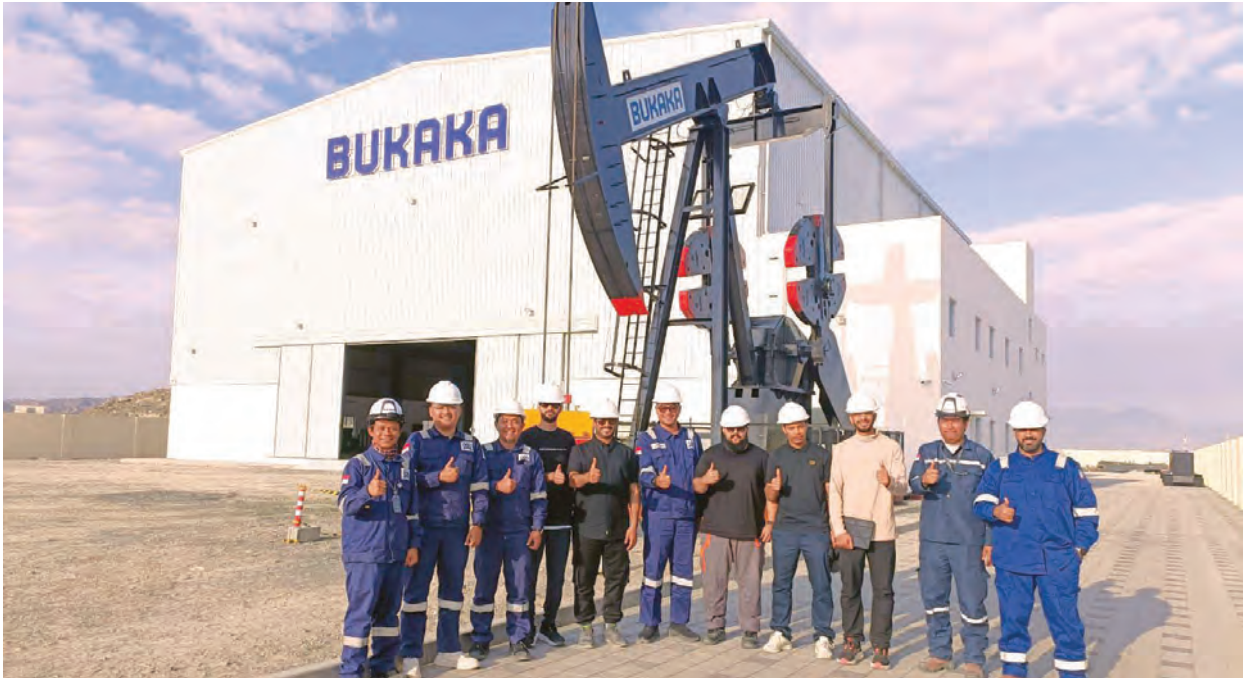
The workshop is positioned as a strategic hub for assembly, testing and future manufacturing of oilfield equipment in Oman.
