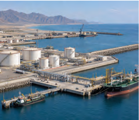
Phase 1 targets around 200,000 tonnes per month of capacity, which is equivalent to 2.4 million tonnes annually (Image for illustration only).
