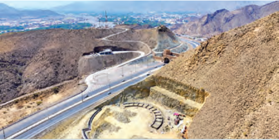
The project is part of a series of development projects presently underway in the Wilayat of Al Rustaq.
